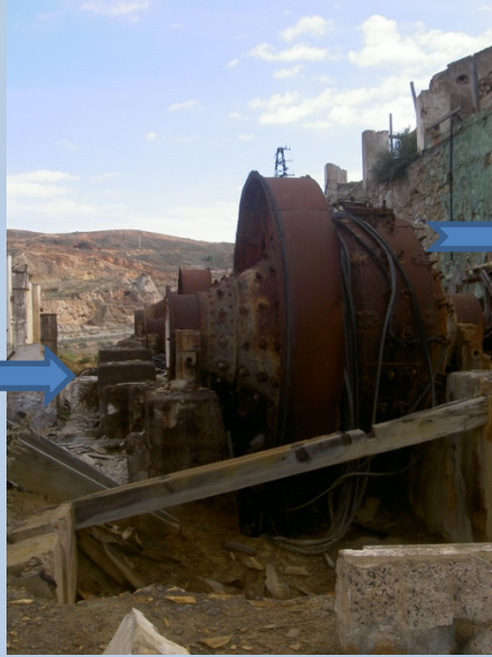
Crushing and grinding the ore to a fine size
